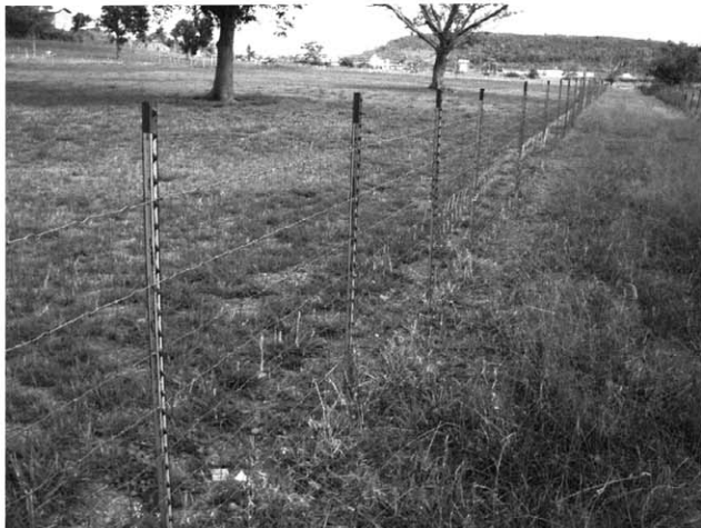
Figure 1. Wire fence supported by metal posts. Fence is attached to the posts by metal clips after the posts are pounded into the ground.
