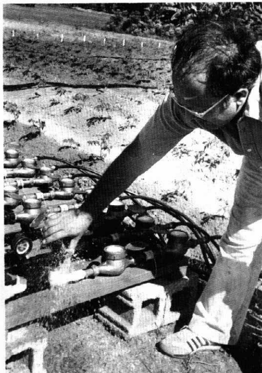
Checking water pressure regulator on irrigation system.
