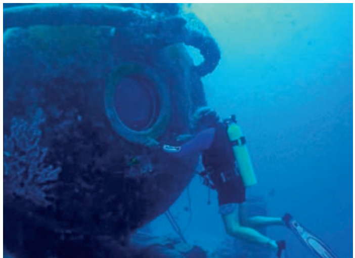
Figure 22. Scuba diver cleans marine growth off of NOAA's Aquarius, an underwater laboratory located in 64 ft. of water at the base of a coral reef in the Florida Keys National Marine Sanctuary. Aquarius provides a special diving capability, called saturation diving, which allows scientists to work out on the reef up to nine hours a day, compared to one hour if they had to work from the surface. Photo credit: NOAA's Undersea Research Program Center at the University of North Carolina Wilmington.
