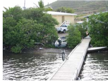
DFW/STT boat dock that needs maintenance dredging
