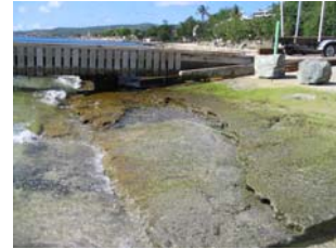
View of ramp
