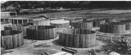
Building additional new fish culture tanks.
