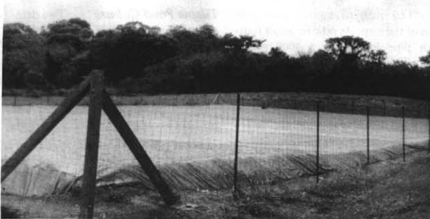
A rainwater catchment to collect and store rainwater from a 100 X 200 foot tarp can collect more than 400,000 gallons of rainwater annually.
